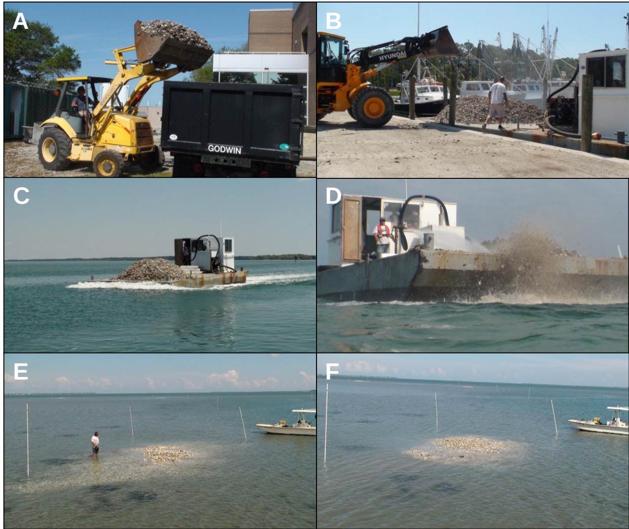
Figure 7. Examples of large reef building activities with assistance from the North Carolina Division of Marine Fisheries. A – loading shell for the trip from IMS to the Harkers Island harbor staging area. B – Captain Thomas “Ger” Hardin directing the loading of shell onto the DMF barge. C – Barge loaded with 300 bushels of oyster shell headed to Middle Marsh. D – DMF technician Michael Jordan using a water cannon to blow shell off of the barge. E – Commercial fisherman Adam Tyler (project participant) looking over a 300 bushel shell pile before shaping. F – Roughly “shaped” large oyster reef, which was fine shaped after the picture was taken.
