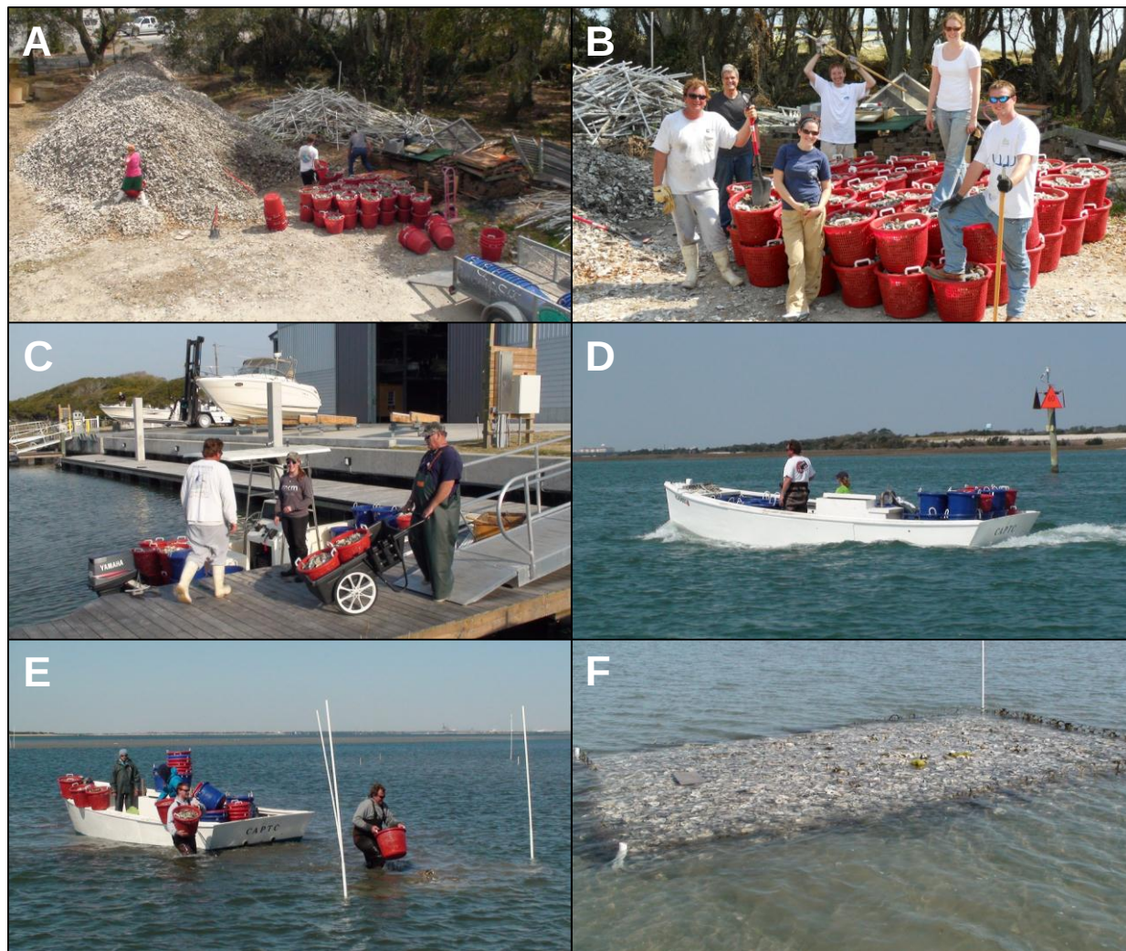
Figure 6. A – digging into the IMS oyster shell pile for small reef building. B – some of the small reef building crew. C – moving baskets of shell from trucks to boats. 1 D – fisherman Adam Tyler and IMS student Sara Coleman taking shell to a reef building site. E – unloading 60 bushels of oyster shell on a small reef plot. F – completed “shaped” small oyster reef.
