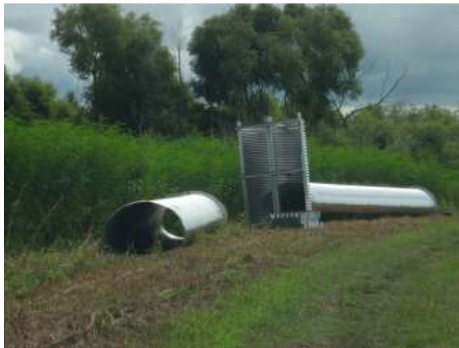
Water Control Structure (WCS) staged and ready for installation.
