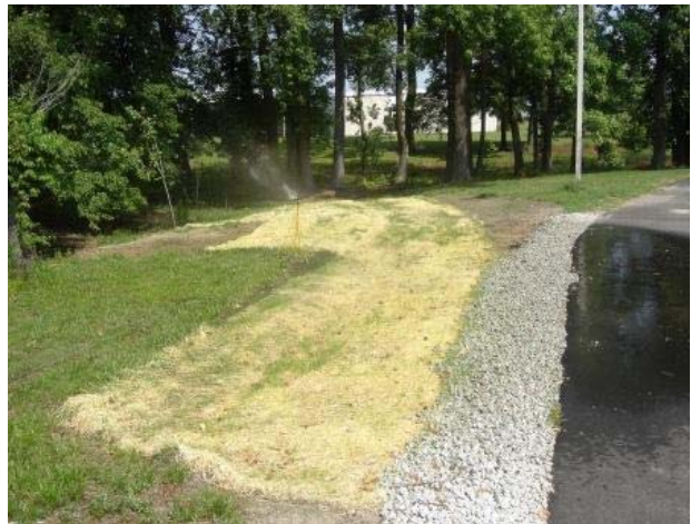
Installation of Grassed Swale for Infiltration
