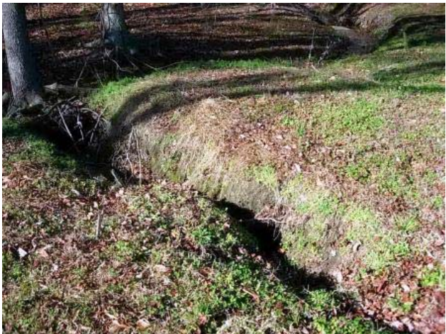
Erosion at Bus Parking Lot (before)
