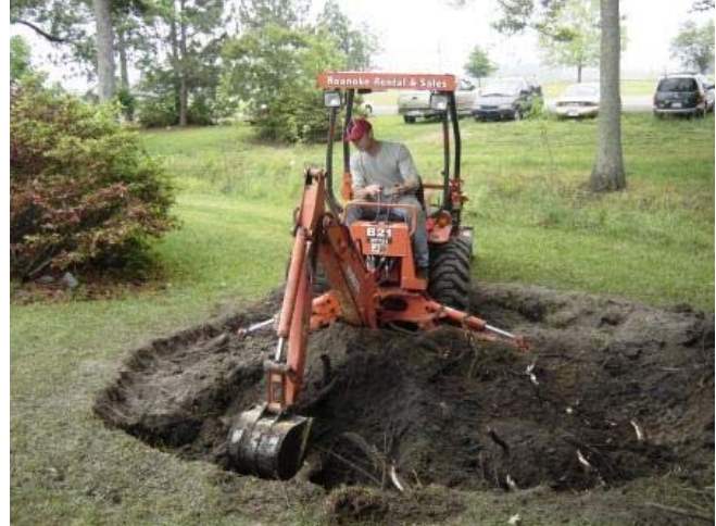
Mitch Woodward of Cooperative Extension excavates rain a rain garden at Vocational Agriculture Building
