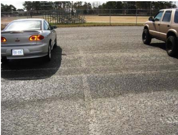
Traditional Asphalt Pavement (before)
