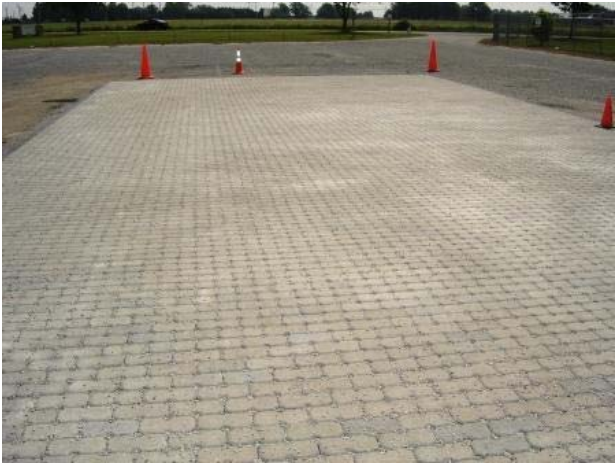
Permeable Pavement Installation
