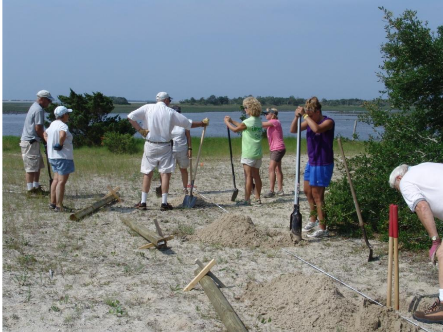
Volunteers installing fence posts on SW side of project site.
