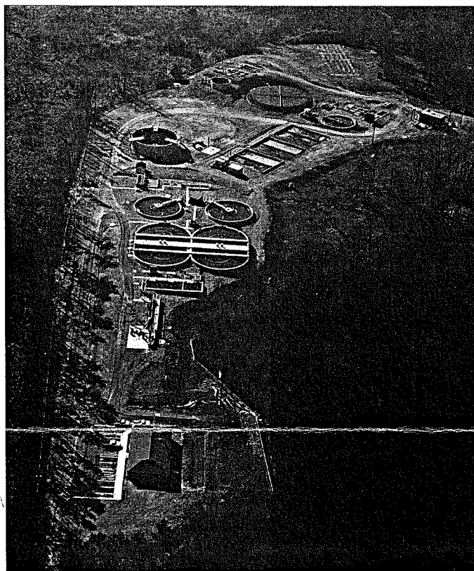
The totally biological BioDenipho® nutrient removal process used at the Tar River Wastewater Reclamation Facility reduces plant energy costs by 40 percent, requires minimal maintenance after four years of operation.
