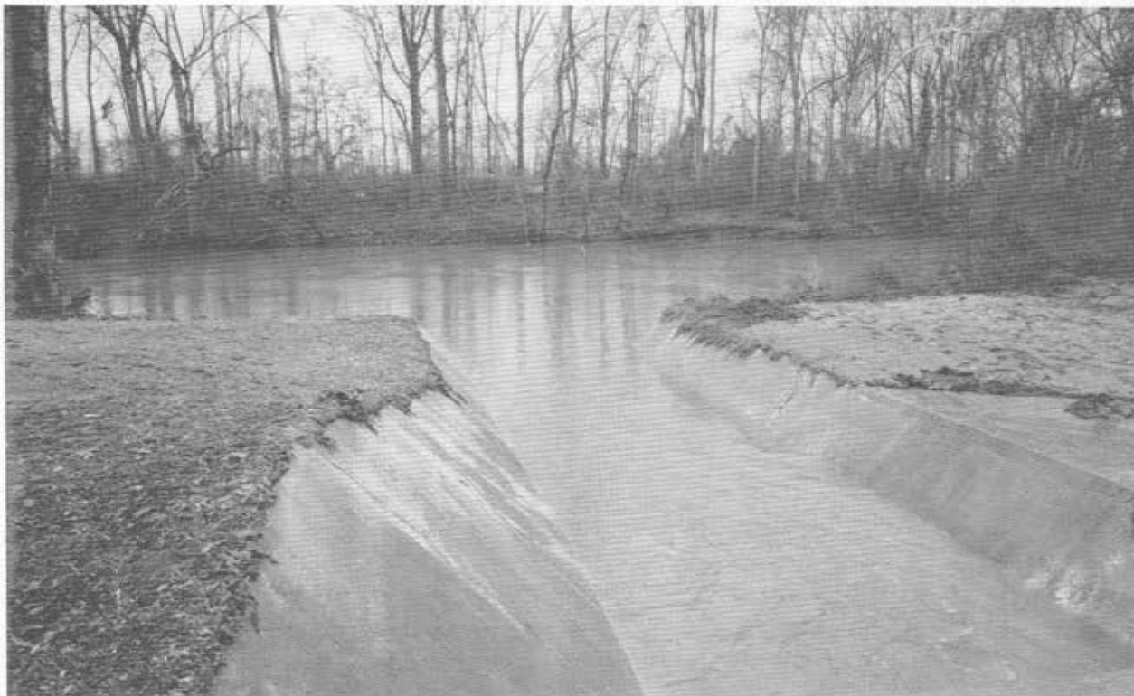
Outfall from Rocky Mount Municipal Wastewater Treatment Plant. (Photo: P. Nurnberg)
