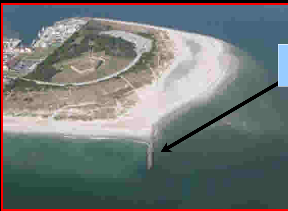
BEAUFORT INLET TERMINAL GROIN AT FORT MACON
