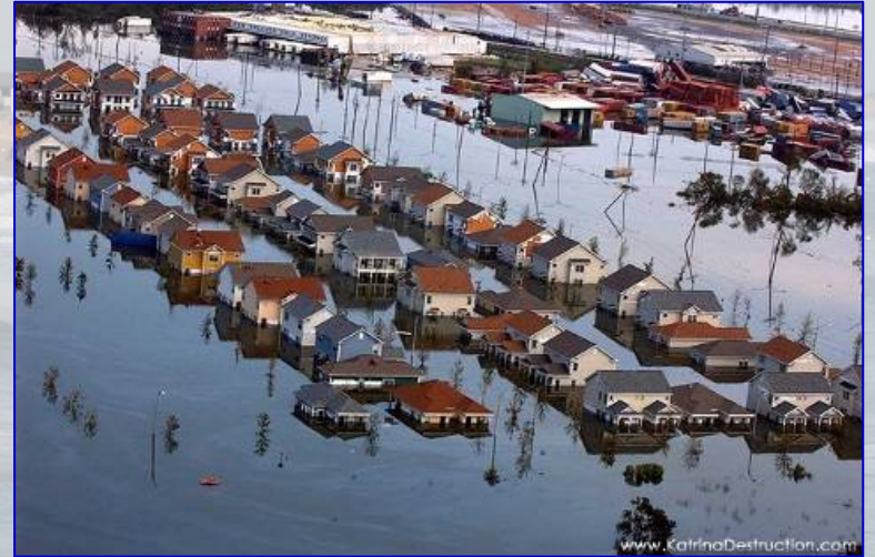
2005 Hurricane Season: Inundation/Flooding
