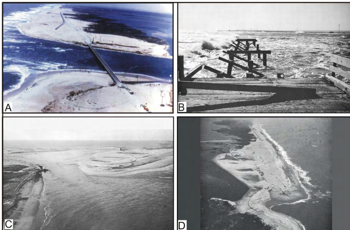
Figure 2-6. A four-part photo series shows the history of Buxton Inlet which opened in the Ash Wednesday Nor'east storm in March 1962. Panel A. An oblique aerial photograph looking south shows the active inlet with a wooden N.C. Hwy. 12 bridge across it. Photograph is by Cape Hatteras National Seashore personnel. Panel B. A nor'east storm in early December 1962 took most of the bridge out. Panel C. An oblique aerial photo looking west was taken on January 29, 1963 and shows the dredge pumping sand from the sound side into the inlet. Panel D. An oblique aerial photo looking north was taken on February 21, 1963 when the inlet was finally closed. Photographs in Panels B, C, and D are from the U.S. Army Corps of Engineers (1963).
