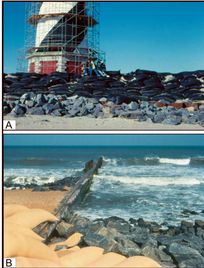
Figure 1-32. Panels A and B. Photographs of the extensive effort to protect the Cape Hatteras Lighthouse from the encroaching Atlantic Ocean with massive hardened structures. These photos show a steel bulkhead, a steel groin, several rock revetments, and many layers of sand bags that have been used over decades in desperate attempts to “hold the line.” Photographs are by S. Riggs.
