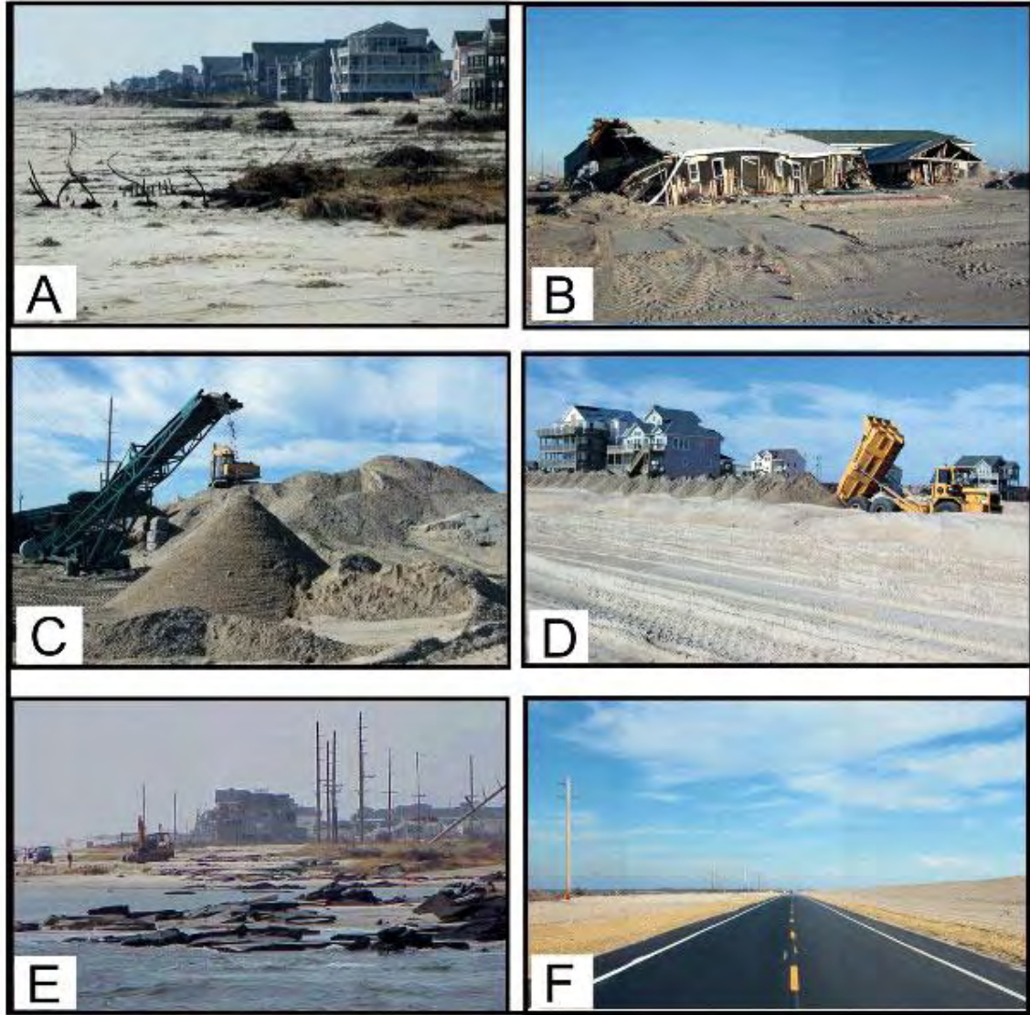
Figure 1-28. Post-Hurricane Isabel (2003) photographs show the damage in Hatteras Village and the newly opened and quickly closed Isabel Inlet. Panel A. Storm surge and overwash destroyed large segments of the barrier-dune ridge. Panel B. This oceanfront motel was destroyed when the barrier-dune ridge was breached by the storm surge. Panel C. This expensive process cleans the debris from overwash sand for use in building the new barrier dune-ridge. Panel D. A new barrier-dune ridge is being constructed in front of the destroyed motels. Panel E. Remnants of N.C. Hwy. 12 pavement within Isabel Inlet. Panel F. This photograph depicts the infilled Isabel Inlet, reconstructed N.C. Hwy. 12, and rebuilt barrier-dune ridge. Photographs are by S.Riggs.
