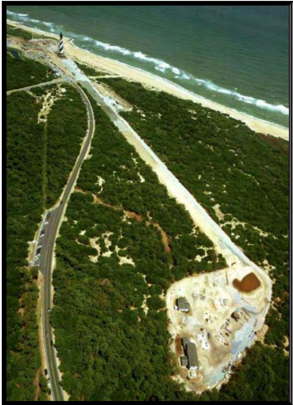
Figure 1-33. Cape Hatteras Lighthouse is being prepared for its move from the old threatened site adjacent to the rapidly eroding shoreline to a new inland site. Photograph is by the N.C. Department of Transportation.
