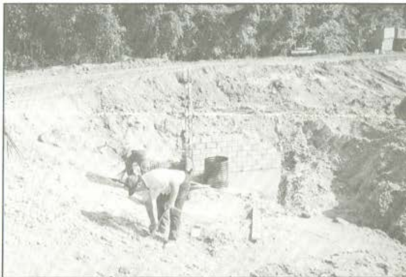
D.5. - D.8. Clockwise from top left: Public Works employees constructing concrete spillway; installation of riser structure and pond outlet discharge piping; site preparation for headwall and pipe installation.
