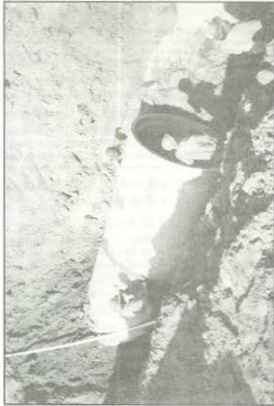
D.9. - D.12. Clockwise from top left: Drop inlet under construction; installation of pond inlet discharge pipe.
