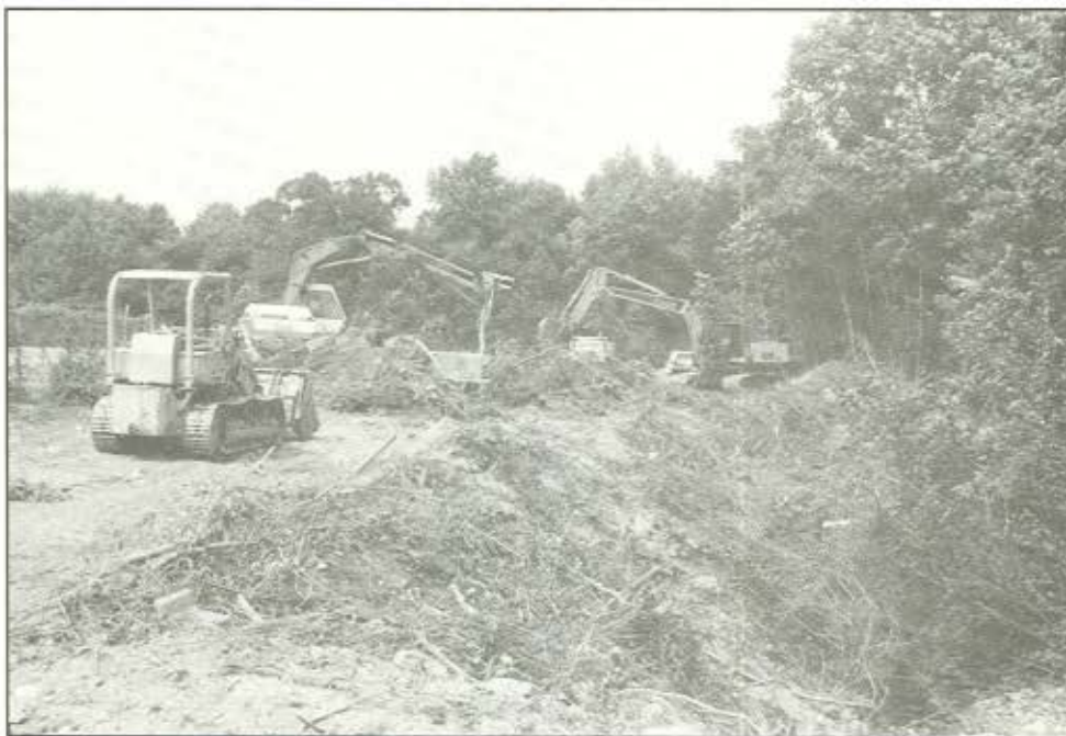
D.4. Land-clearing activities at Moyewood Ditch.
