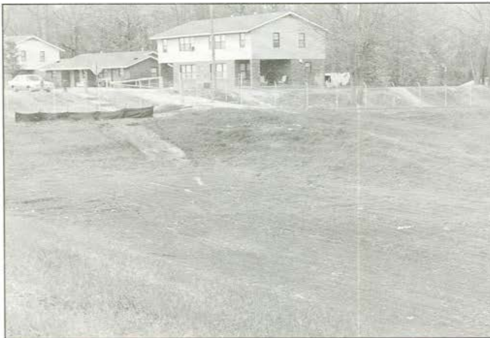
D.17. West Conley entrance to detention basin.
