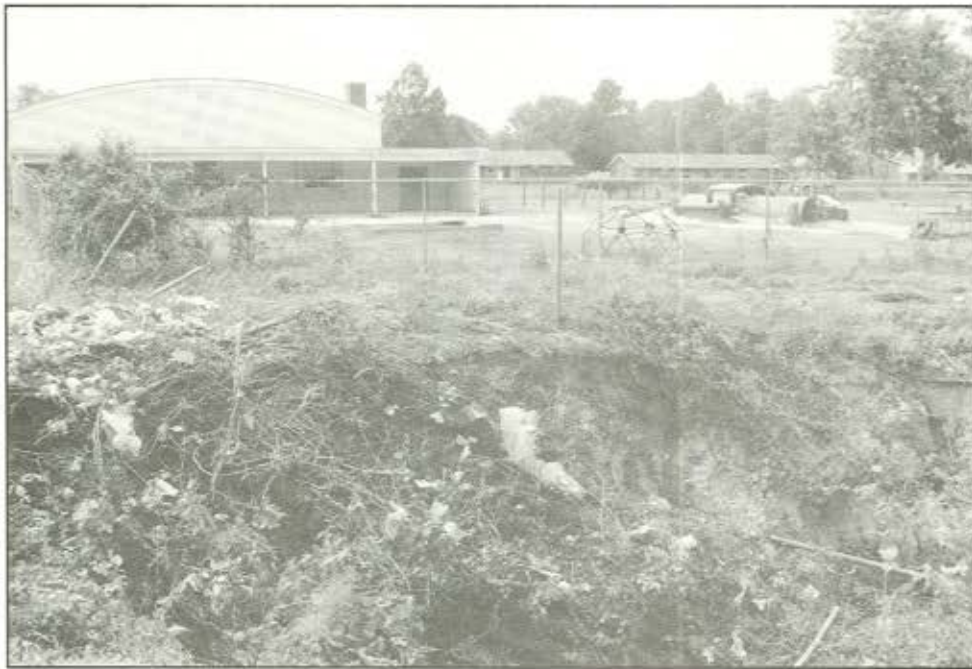
D.3. Moyewood Ditch. Daycare Center is in background.
