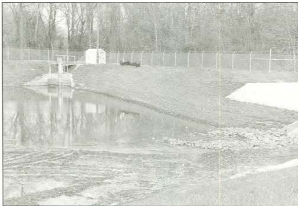
D.23. Storage shed behind outlet structure contains ICMR sampling equipment. Note outdoor lightpole. Inlet discharge pipe, trapezoidal spillway to right.
