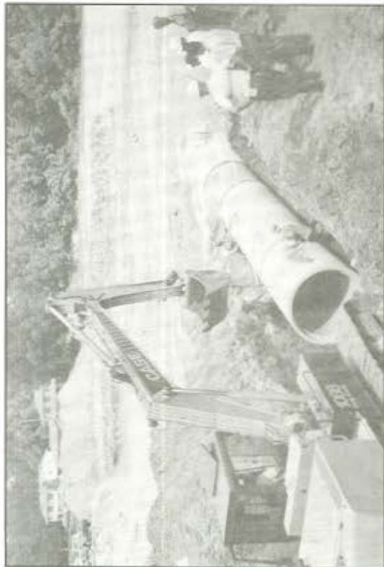
D.9. - D.12. Clockwise from top left: Drop inlet under construction; installation of pond inlet discharge pipe.
