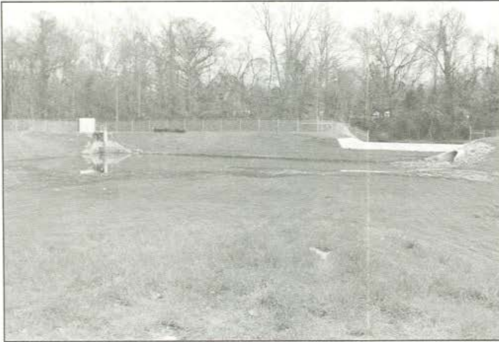
D.16. View from West Conley entrance. Outlet structure to left. Spillway, inlet pipe at right.
