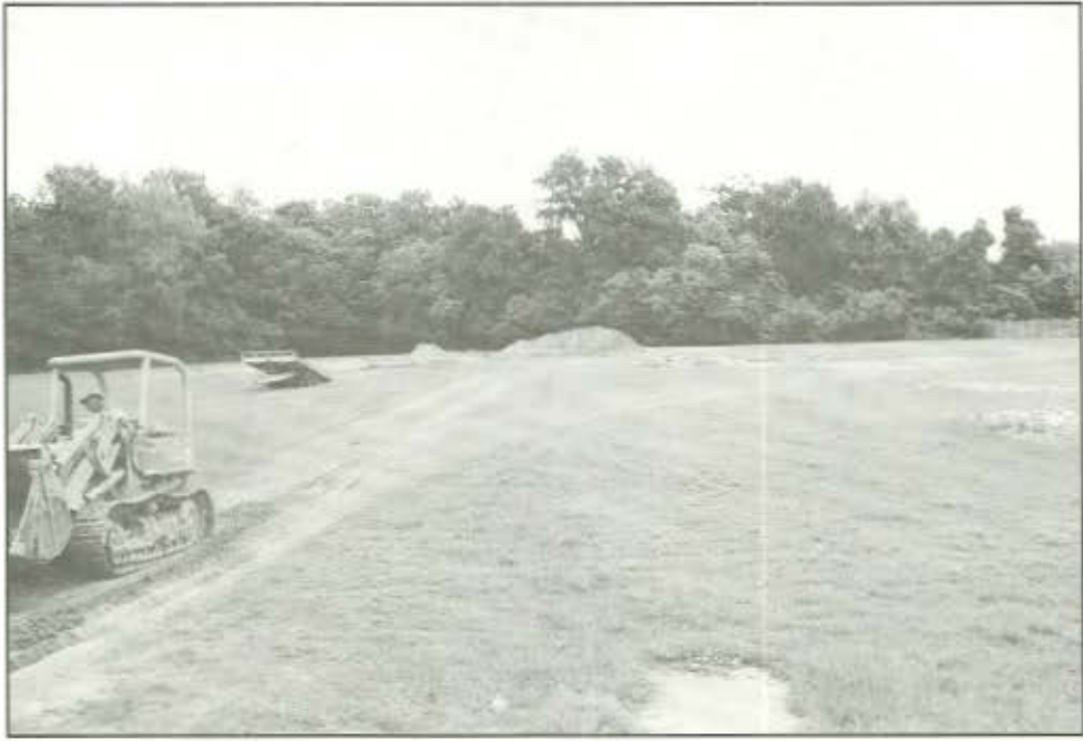
D.1. Excavation of detention pond begins.
