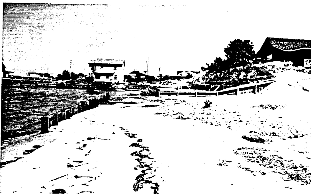
Figure 8b. After breakwater construction. Beach width increased due to March storm.
