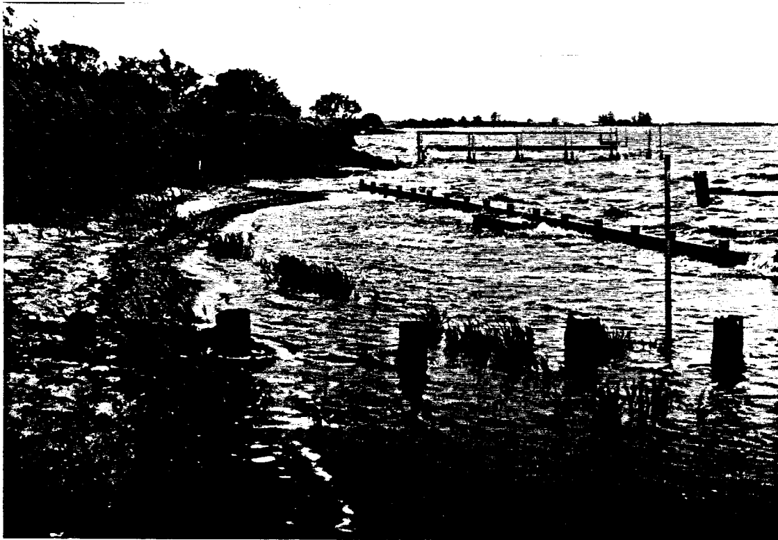
Figure 9b. Two years after construction and planting.
