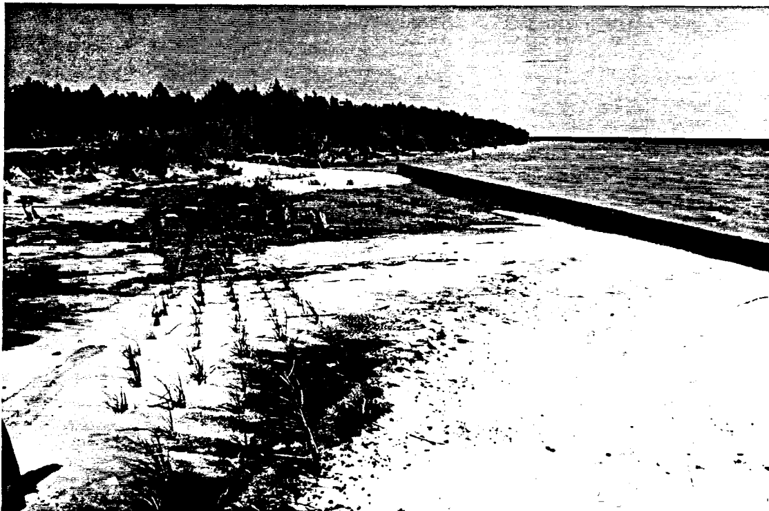
Figure 11. Site 11, one year after breakwater construction.
